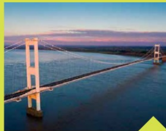
M48 Severn Bridge
